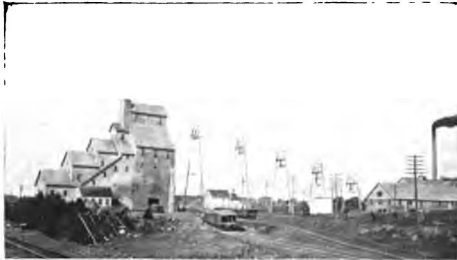
A. MESNARD SHAFT, QUINCY MINE.
